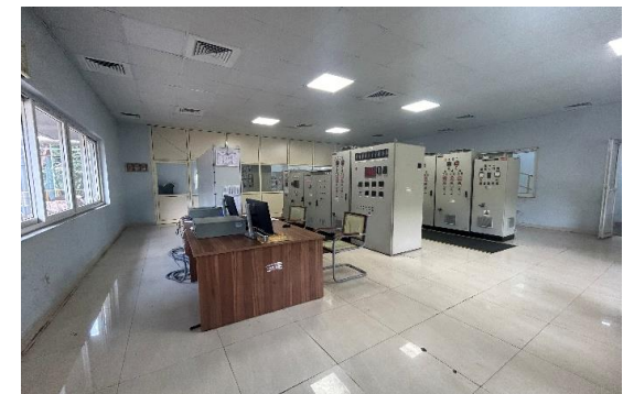
Thermax Boiler design for Bio mass
